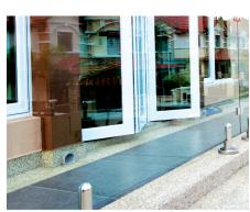
Our Frameless Glass Clamp Railing System provides an almost invisible "frameless" look. No vertical posts are used between the panels of glass; they are solely supported from the bottom by high strength stainless steel clamps.
