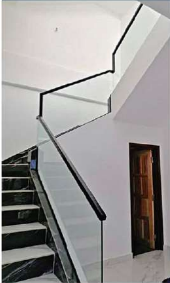
Embedded Aluminium U Channel
