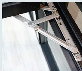
Support Bar Hinge SUS304 Stainless Steel
